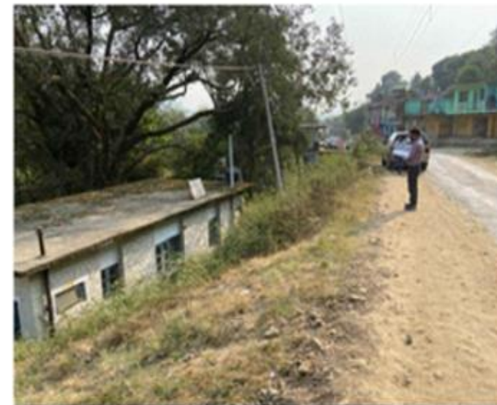
PRESENT SITE PHOTOGRAPH AT CH 4+515
