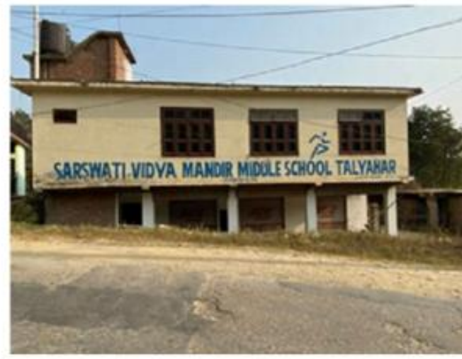
PRESENT SITE PHOTOGRAPH AT CH.4+773
