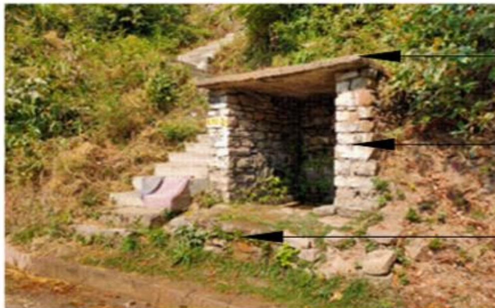
RENOVATION OF NATURAL WATER SOURCE AT CH 10+416.
