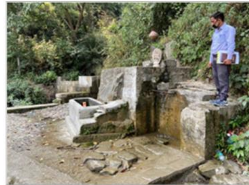
PRESENT SITE PHOTOGRAPH AT CH 3+700
