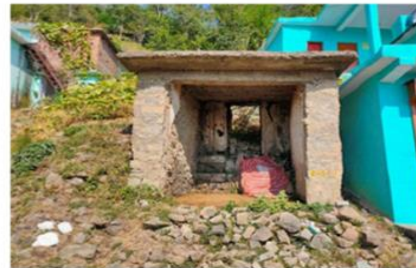
PRESENT SITE PHOTOGRAPH AT CH 24+218
