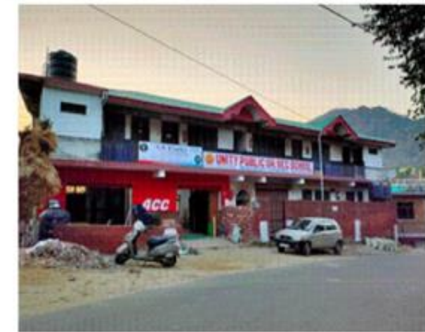
PRESENT SITE PHOTOGRAPH AT CH.22+545
