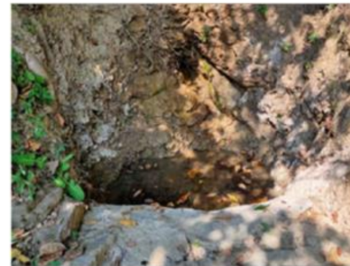
PRESENT SITE PHOTOGRAPH AT CH 12+482
