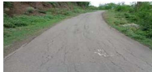
Road Condition @Km 14+420
