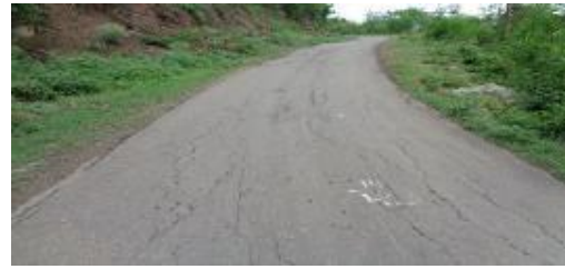
Road Condition @Km 14+420
