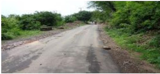
Road Condition @Km 11+550
