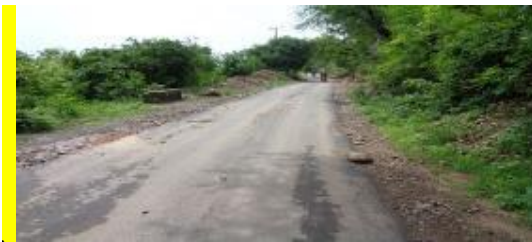
Road Condition @Km 11+550
