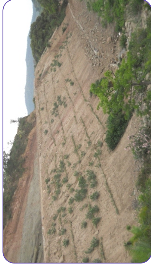
(Bamboo Crib Wall Formation : Barsar-Jahu Road, Chainage 67+200)
