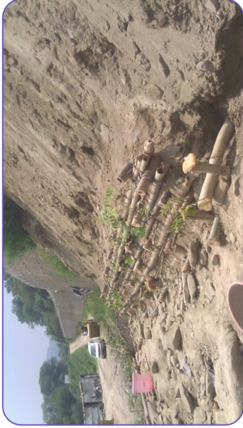
(Bamboo Crib Wall Formation : Barsar-Jahu Road, Chainage 67+200)
