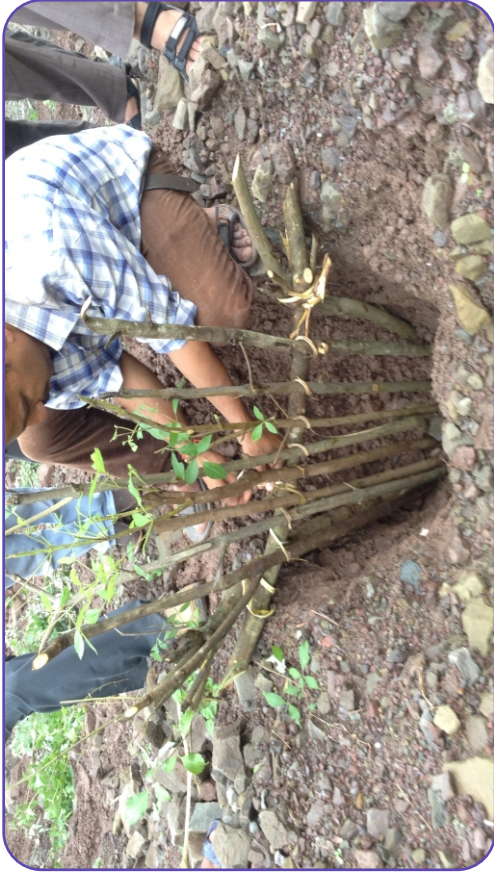
(Construction of Palisade : Kumarhatti-Nahan Road, Chainage 59+620)
