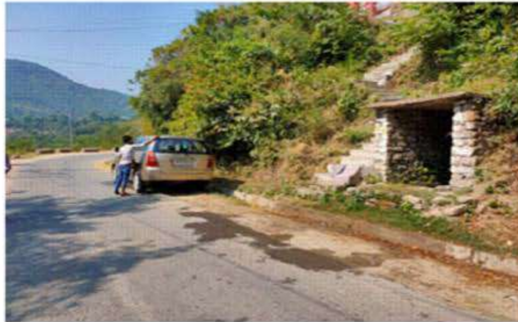
PRESENT SITE PHOTOGRAPH AT CH 10+416
