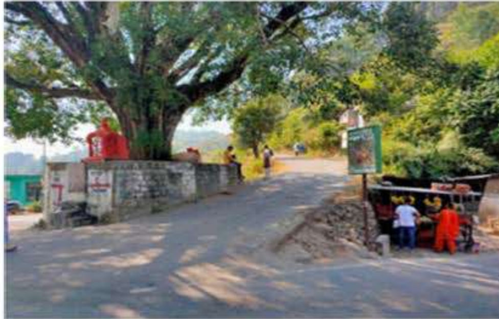
PRESENT SITE PHOTOGRAPH AT CH 28+415
