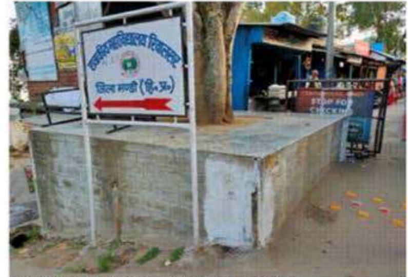
PRESENT SITE PHOTOGRAPH AT CH 22+997
