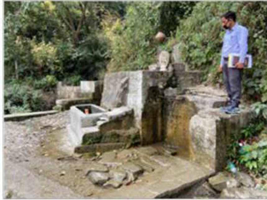
PRESENT SITE PHOTOGRAPH AT CH 3+700
