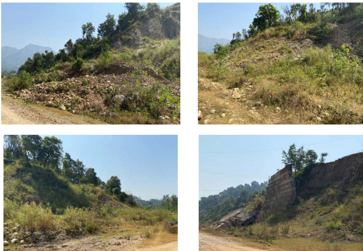
Figure 7-12: Landslide Prone locations along Project Road (Between Ch 1+45 to 2+74)
