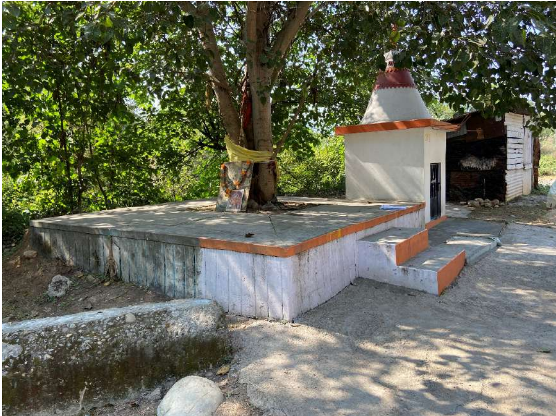
Figure 6-2: Partially Impacted Religious Structure at Ch 1+052
