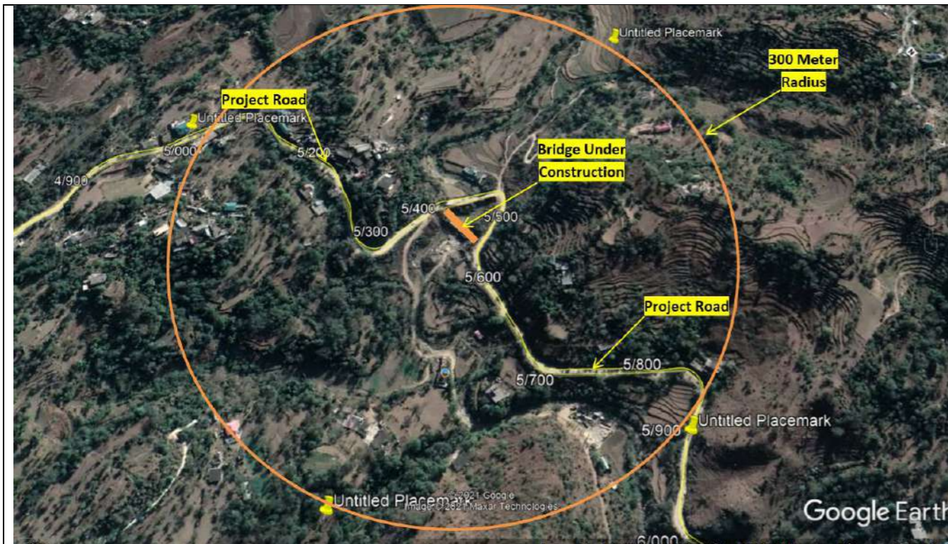
Minor Bridge under Construction at existing Ch. 5+820/ Design Ch 5+719 Coordinates: 31°40'24.74" N/ 76°54'29.48" E
