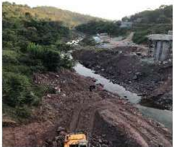
Riverbed used as Access Road
