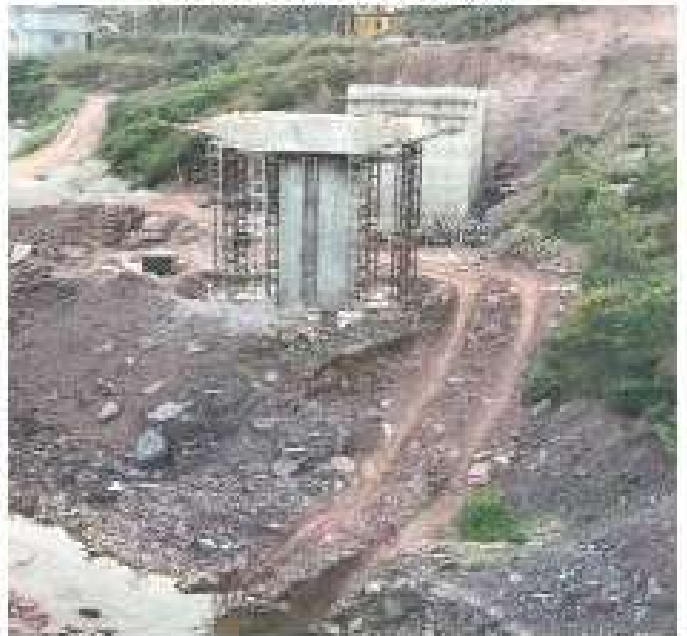
Bridge Pier Construction on Riverbed
