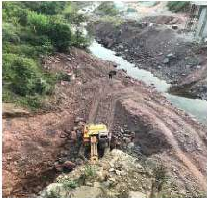
Earth Excavation from Riverbed
