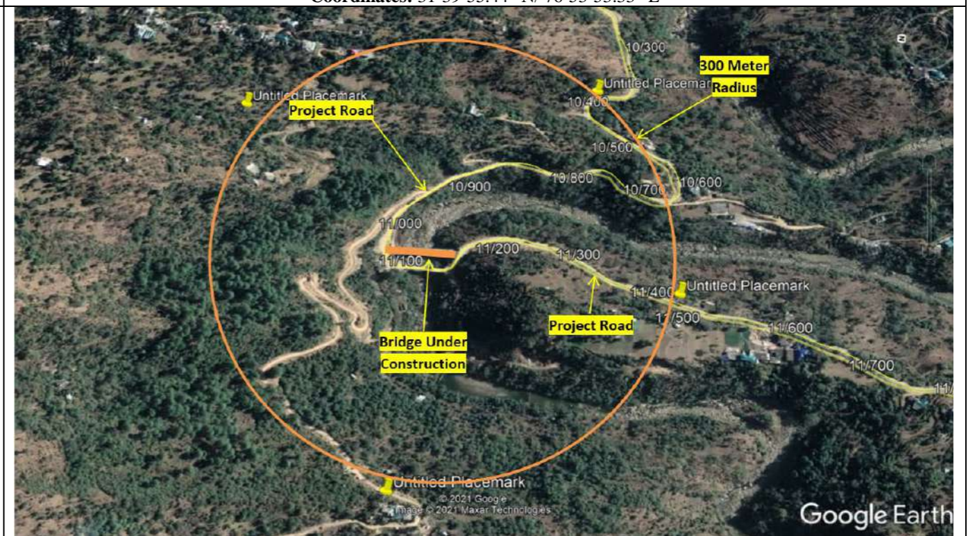
Minor Bridge under Construction at Existing- Ch 11+475/ Design Ch 11+054 Coordinates: 31°39'15.05" N/ 76°52'50.61" E
